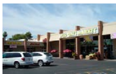
Arcadia Village: Latest acquisition was an Arizona strip mall
